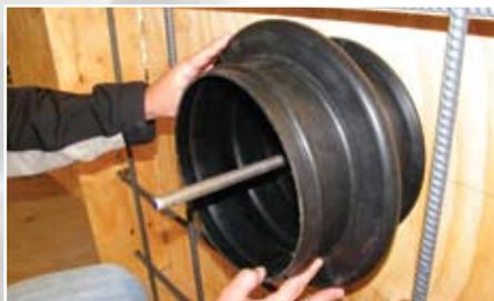
2. Attach INFINITY® wall sleeve to locator cap.
