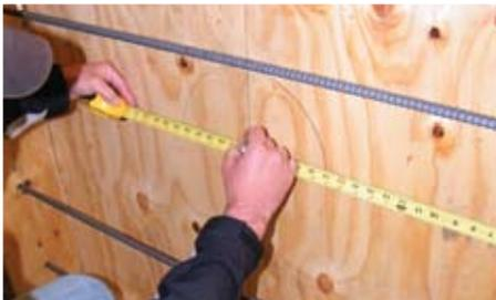
1. Using a tape measure, pull measurements from the horizontal and vertical positions to locate the center of the INFINITY® sleeve.
