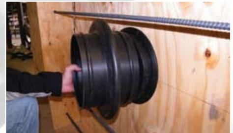
3. Cut the INFINITY® sleeve ¼" longer than the wall thickness. Insert the INFINITY® sleeve over the locator cap.
