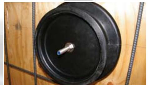
3. Slide second locator cap through (threaded rod\*), use fender washer and fasten nut until locator caps and sleeve is locked in place. Check to make sure sleeve is square to form.
